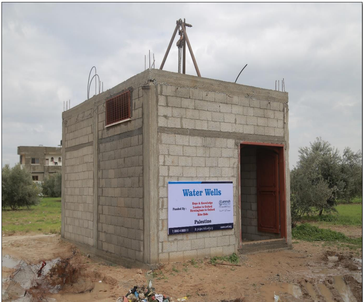
Galvanized Steel Doors and Window Has Completed
