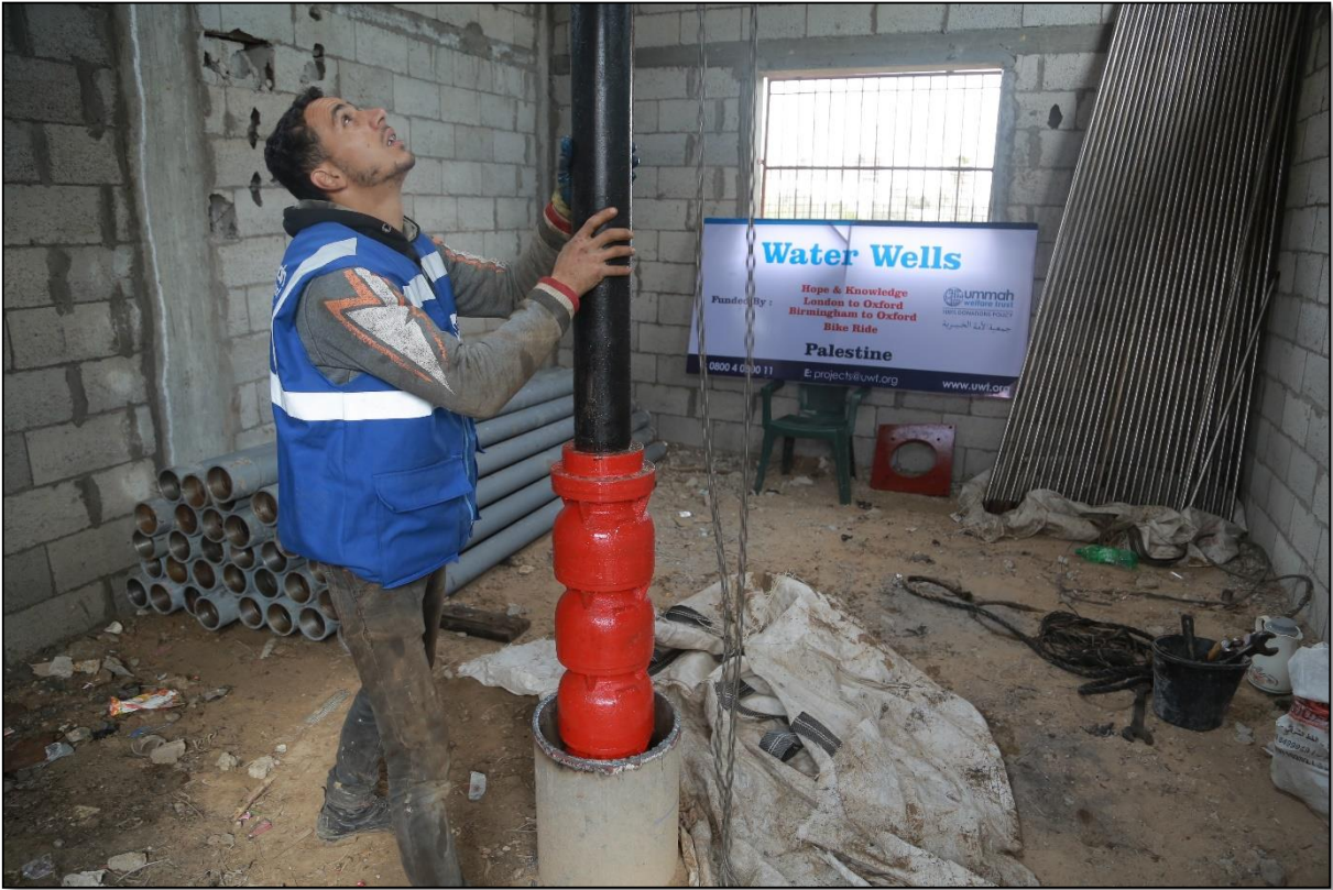
The Pumping Manifold has been installed
