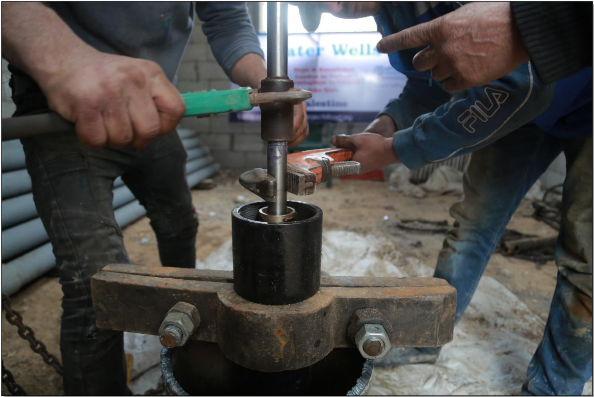
Water pumping unit, chlorine disinfection system completed
