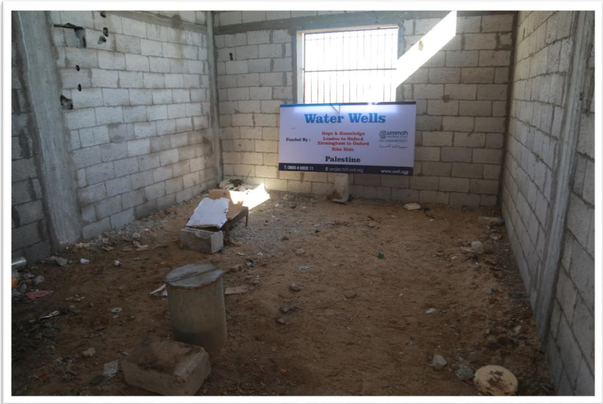
Water pumping & purification building ready to be plastered and painted
